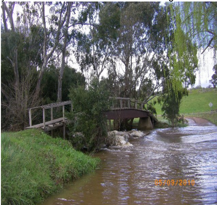
The Bridge over the River Crow – Jones
